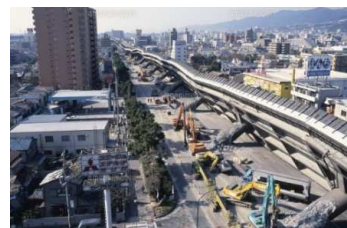
The highway collapsed in the Great Hanshin Earthquake. Our products supported the reconstruction.
