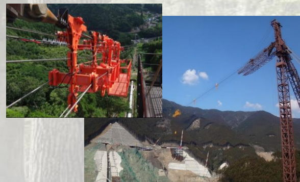
[Cable crane for dam construction and power plants and dams]
